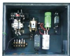
Interior View of MR-G2W
