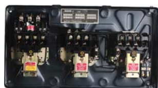
Interior View of MK1 FASD
